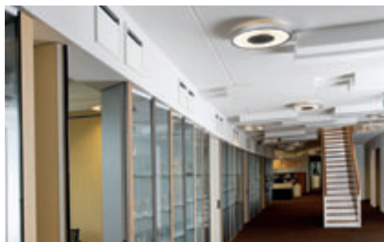
9. Overstroomopeningen hoog in de wand.
